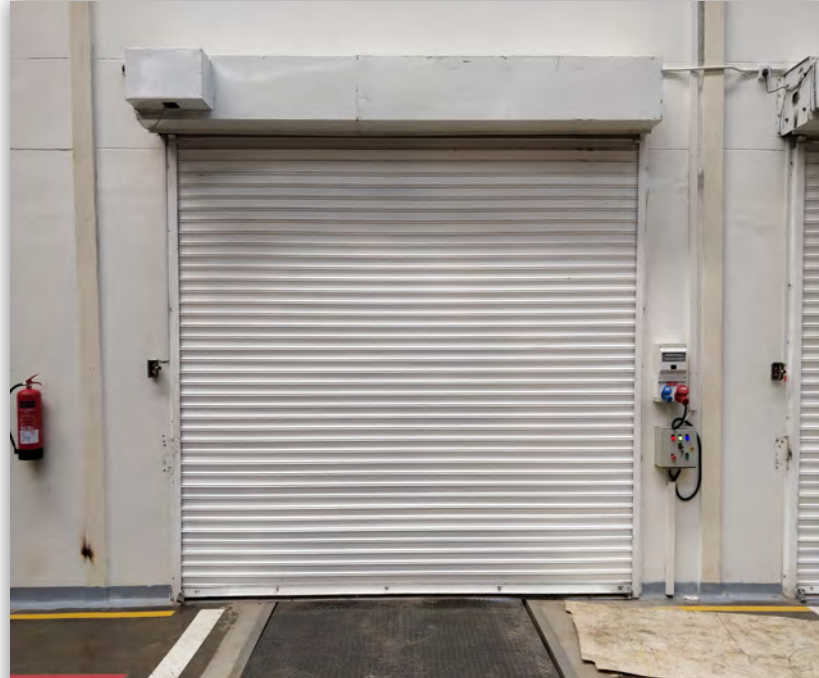
Motorized Roller Shutter
